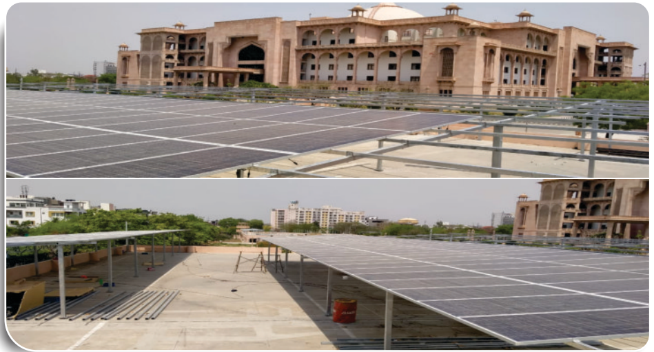
560 kWp Grid Connected Solar Power Plants (Car Port ) under Installation at Rajasthan Vidhansabha , Jaipur
